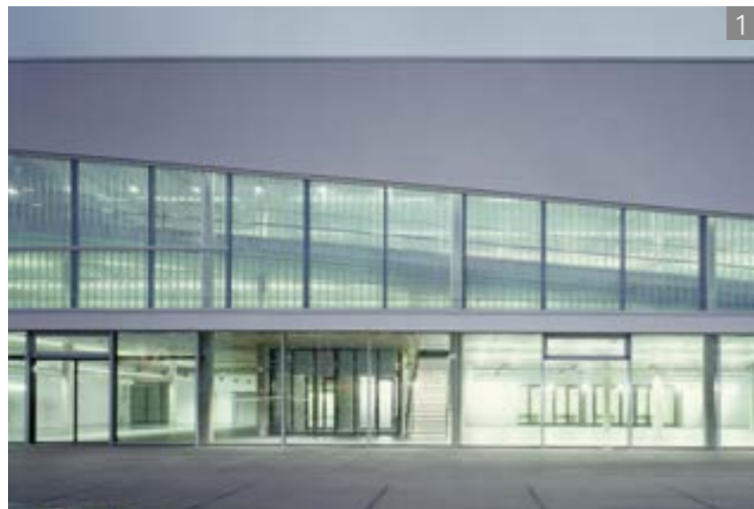
1. BMW Automobile Zentrum: Neubau, Hamburg-Ost | BMW car centre: New building, Hamburg-Ost.
